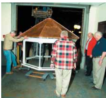
Getting the Lantern Room through the door was tough!
